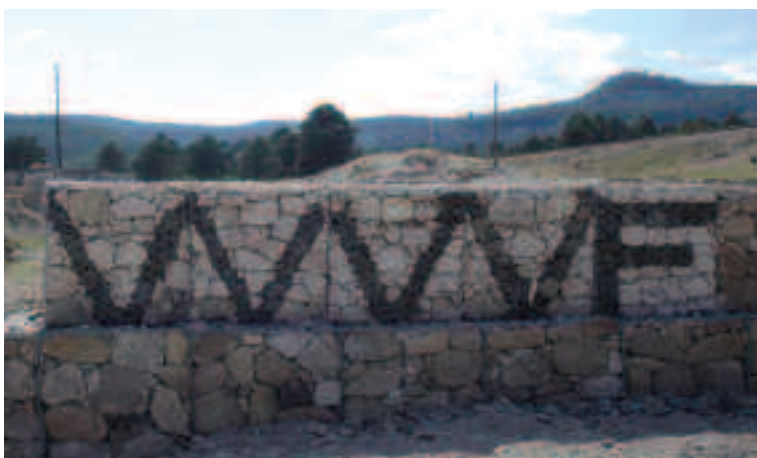
Gabion dam, named after WWF. © WWF / Jenny ZAPATA
