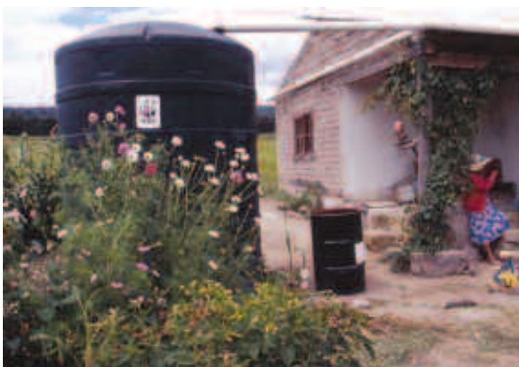
Community rainwater collection system. © WWF / David Lauer READ
