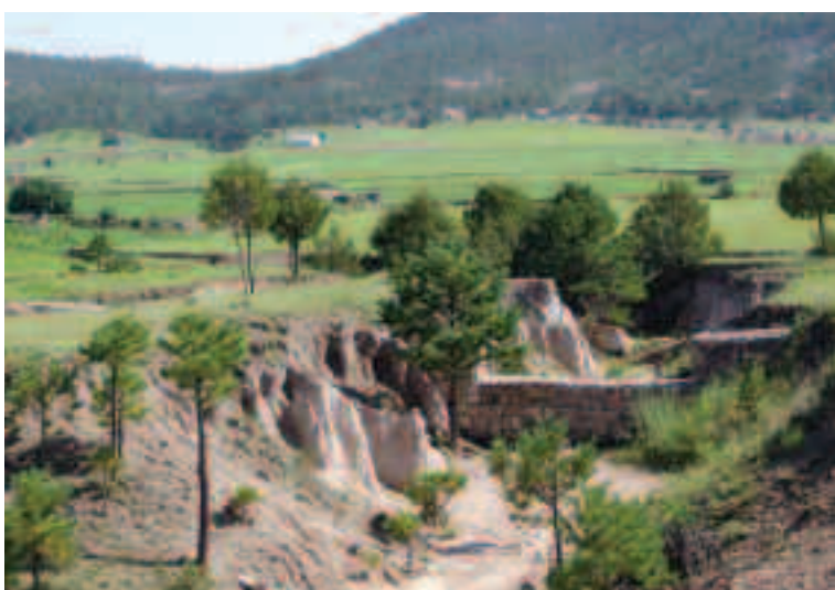
Gabion dam in eroded stream channel. © WWF / Jenny ZAPATA
