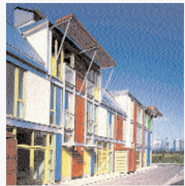
New sustainable homes at the Greenwich Millennium Village.
