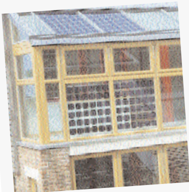
A sustainable home in the London Borough of Sutton.
