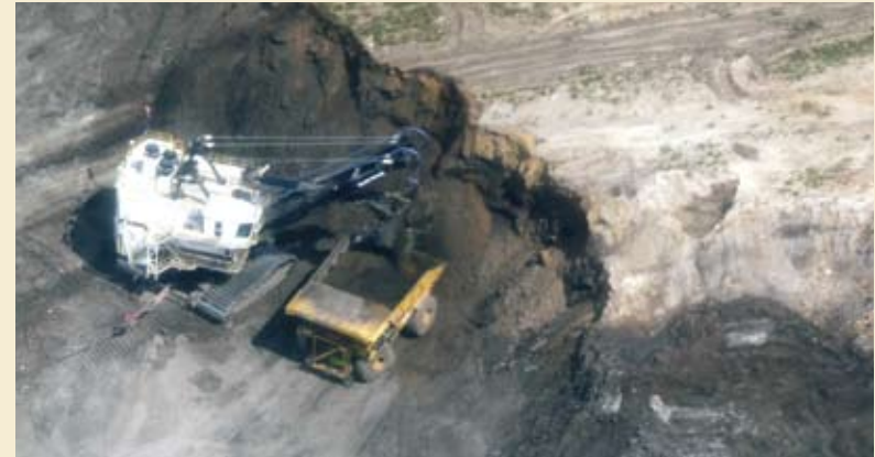
Figure 1.2.1-1 Oil Sands Mining, Photo by David Dodge courtesy of The Pembina Institute, (www.OilSandsWatch.org)
