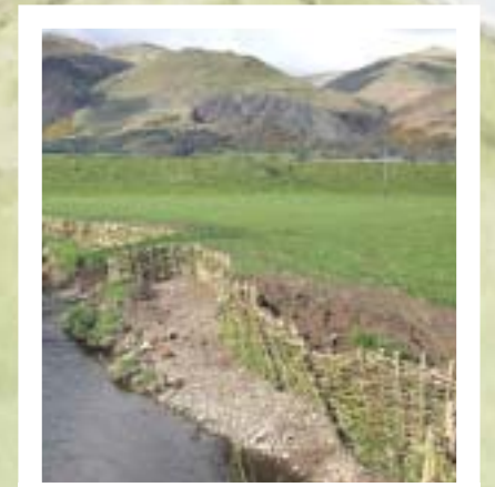
Livestock will be fenced away from the river with willow walls created to prevent bank erosion. Drinking water will be provided for the animals in fields.
