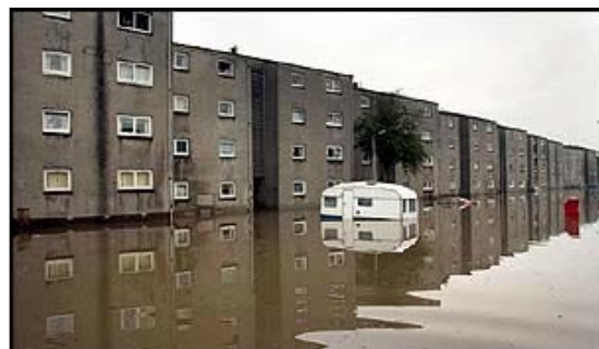
Flooding on a developed floodplain
