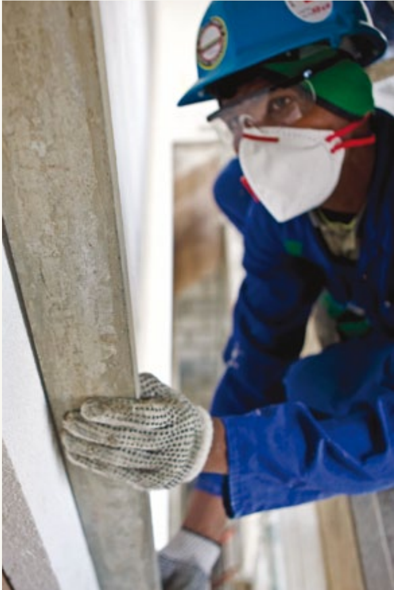
A craftsman glues an insulating panel on to the facade of the East Hotel in Dubai. The building is optimally insulated thanks to BASF's multi-layer SENERGY insulation system. This reduces the energy used to cool the building by 50 percent.
