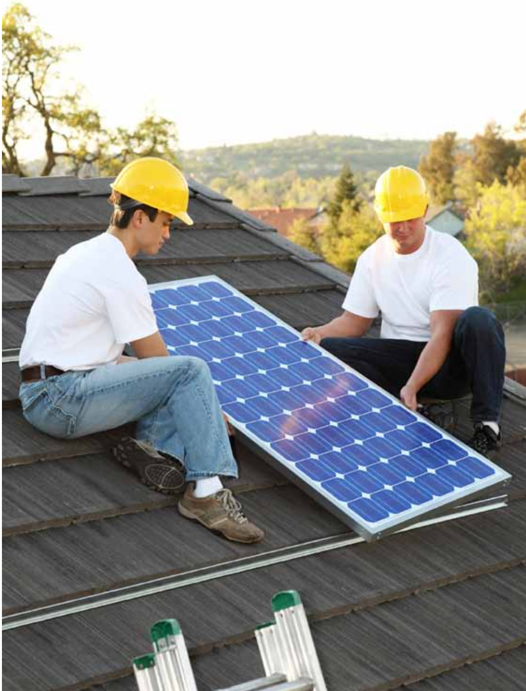
Solar installers on house.
